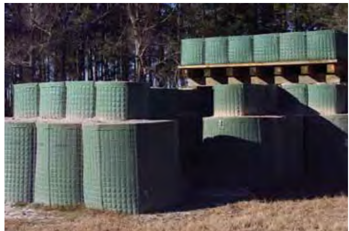
HESCO concertainer revetment for splinter protection.
