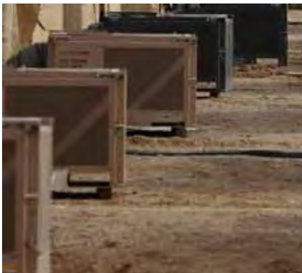
Shut off HVAC.
